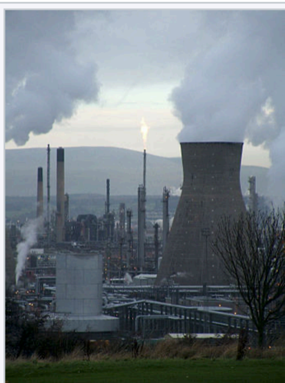
A petrochemical refinery in Grangemouth, Scotland, UK
